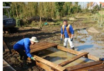
Building the boardwalk
