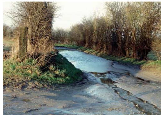
Water and sediment accessing public highways
